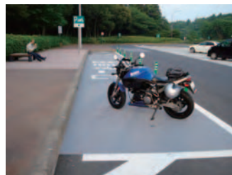
Construction sample for parking lot
