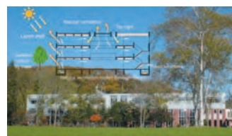
The simple building form, exterior insulation and highly-insulative sash windows
