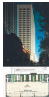
The floors slabs have removable portions, and each floor has two sets of toilets.
