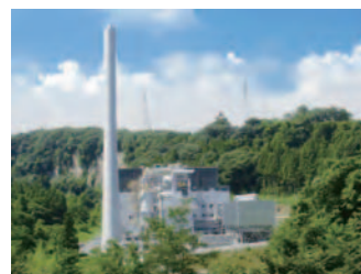
Agatsuma Biomass Power Plant
