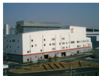
The zero-emission plant at the Sai-no-kuni Resources Recycling Facility
