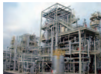
PLA Production Plant
