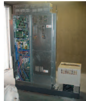
Elevator Control Board Refurbishment Note: Covers are taken off for reference
